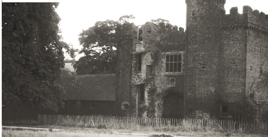
Damage to Lullingstone Gatehouse from V1 of 11/11/1945, here in 1952 before repairs.
