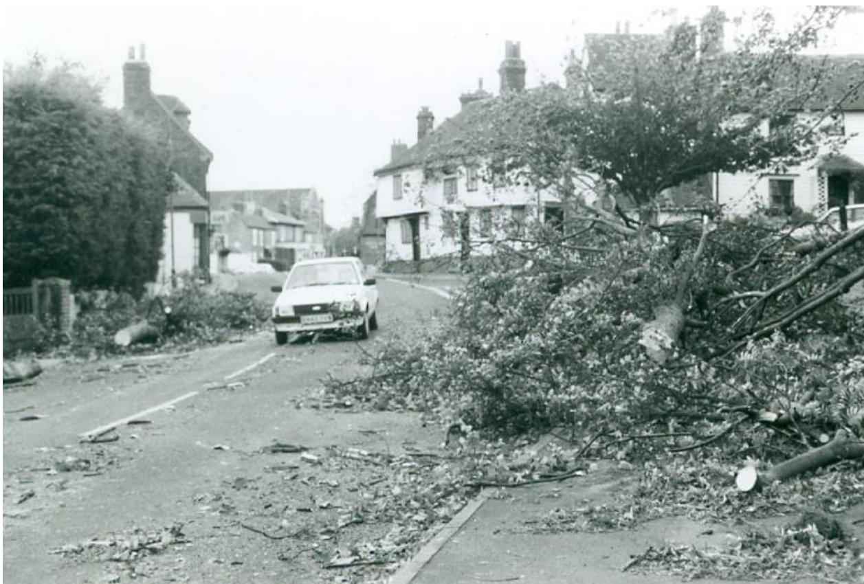
Eynsford High Street looking north from the bottom of Bower Lane. Elizabeth Cottages on right.
